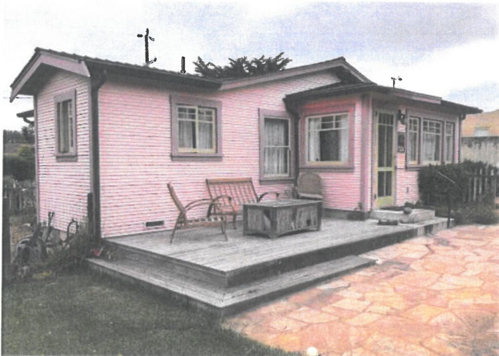
Figure 5: View of Hinshaw-McGovern House with bearing of 48.95 Northeast. Parcel located at 833 Maple St, Pacific Grove, CA 93950, APN: 006-634-050-000.
