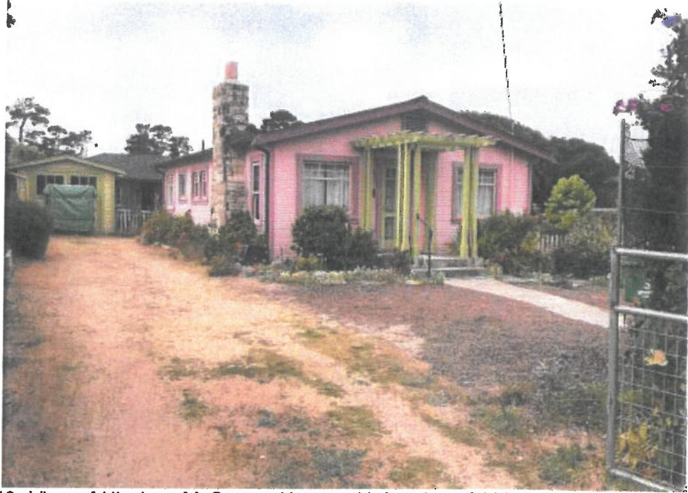
Figure 10: View of Hinshaw-McGovern House with bearing of 208.79 South. Parcel located at 833 Maple St, Pacific Grove, CA 93950, APN: 006-634-050-000.
